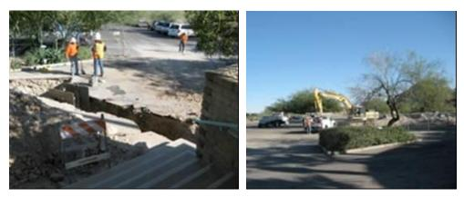
The existing plumbing was completely converted to the Phoenix sewer system on December 29, 2011. The existing septic tanks have been filled with slurry and sealed.
