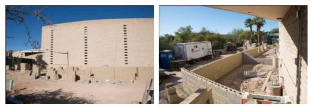
In February, the walls of the new addition reached the top. The walls extend above the roof of the restroom to block vision of the new heating and air conditioning unit. A view down the main hallway shows the four new doorways for the Men's, Women's, and two Family restrooms.
